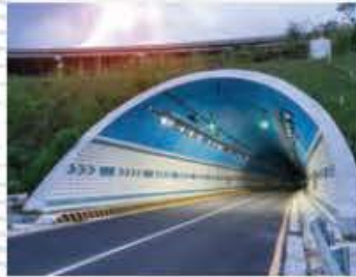
BORIVALI - THANE TUNNEL
