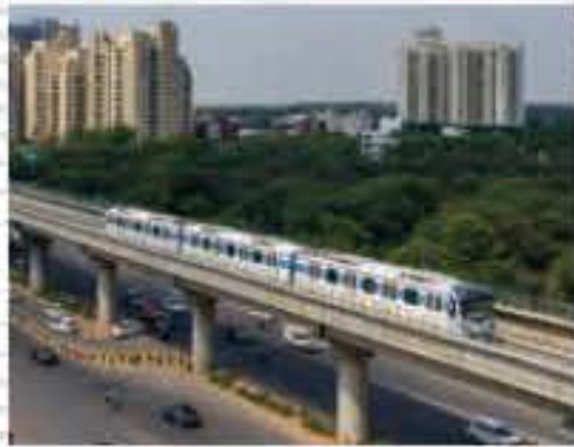
MUMBAI METRO LINE 5
